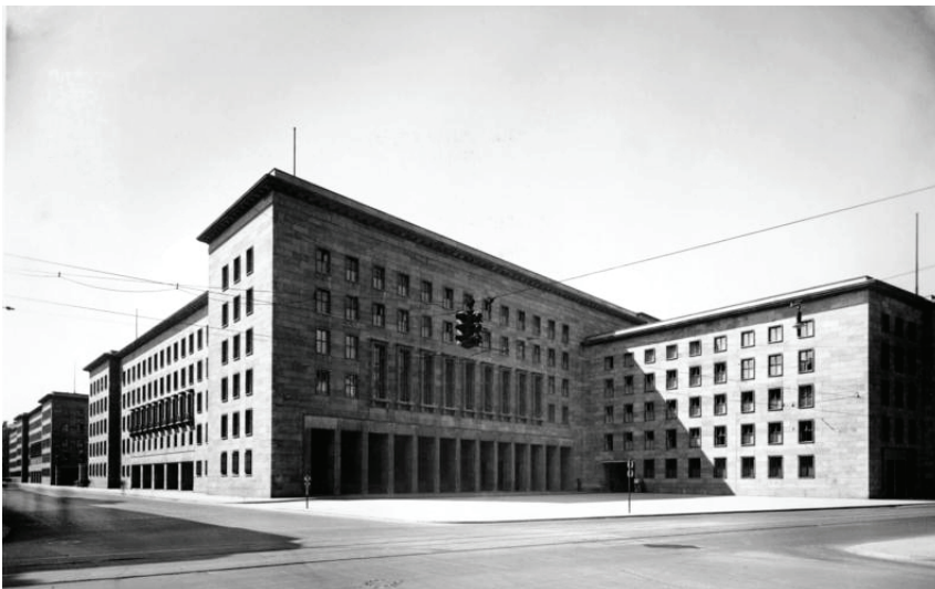
The Air Ministry Building
